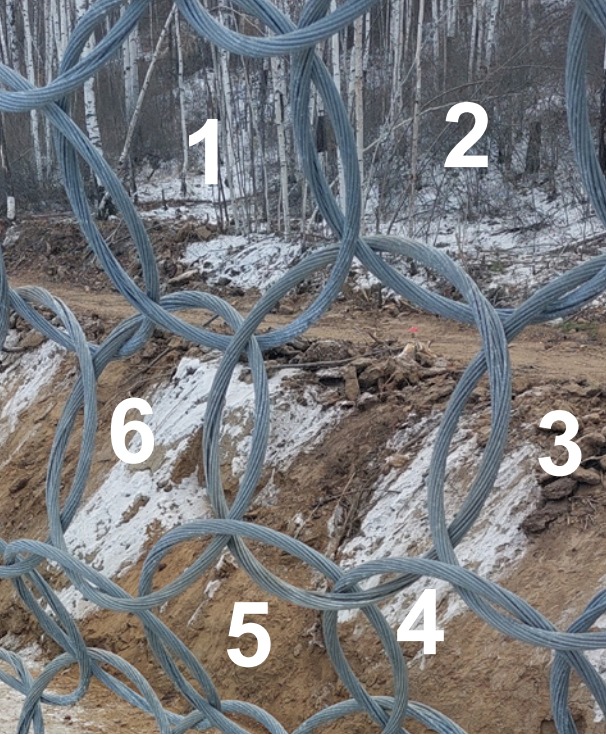
Six-point weaving: each ring is interwoven into six adjacent rings.
